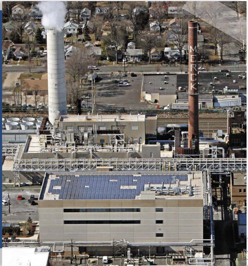
From Solar Electric, LLC
